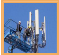
RMWT employees performing mobile communications tower construction
